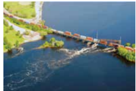
2014 flood year high water under bridge at Ranier 7/14/2014
